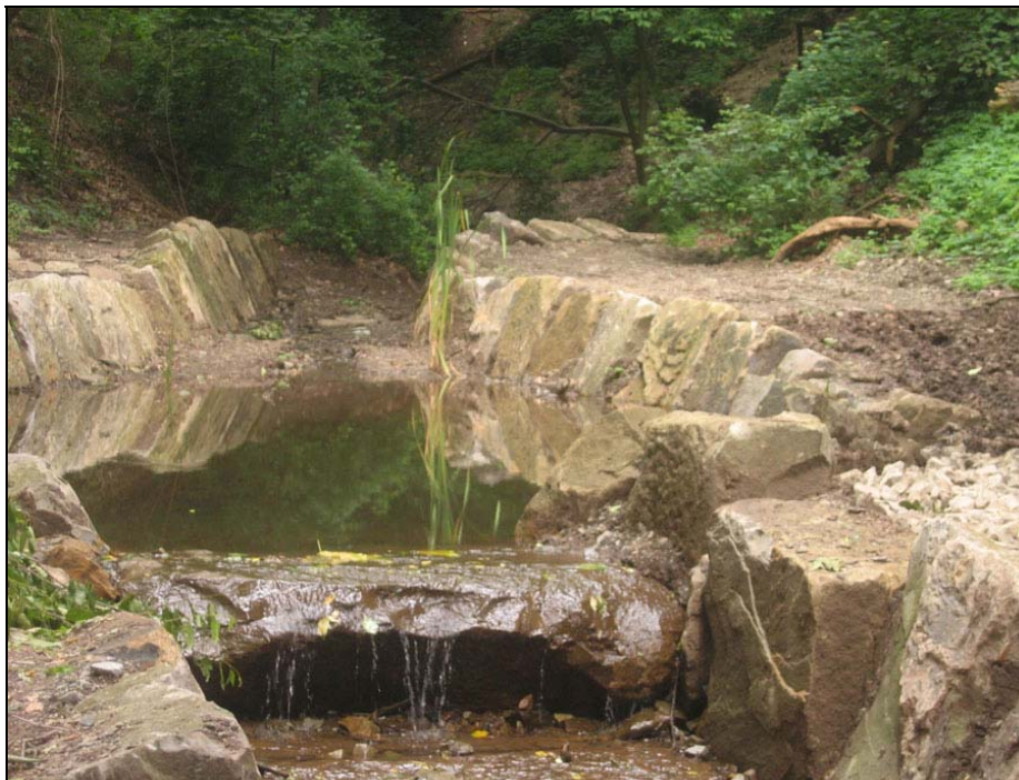
Figure VIII.2 Basin constructed in degraded Phipps Run stream channel, Schenley Park, Pittsburgh, by DPW crews under direction of Pittsburgh parks Conservancy and Heritage Landscapes. (SP-PhippsRunBasin.jpg HL, 2004.)
