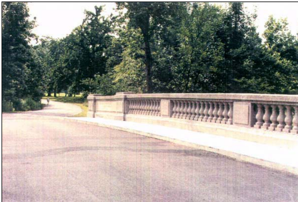
Figure VIII.5 New deck for increased load and original repaired balustrade on Red Creek Bridge, Genesee Valley Park, for Monroe County Parks, Clark Patterson Engineers, Heritage Landscapes preservation consultant. (GVP-red-creek-bridge-deck.jpg, HL, 1997)
